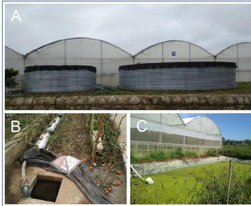
**Figure 2.** Reservoirs in Cascade ReUse Systems (CRUS), namely (A) galvanized steel tanks, (B) underground concrete reservoir and (C) irrigation pond, where drainages originated from fertigation of soilless production are retained to be used for fertigation of soil-grown crops.
